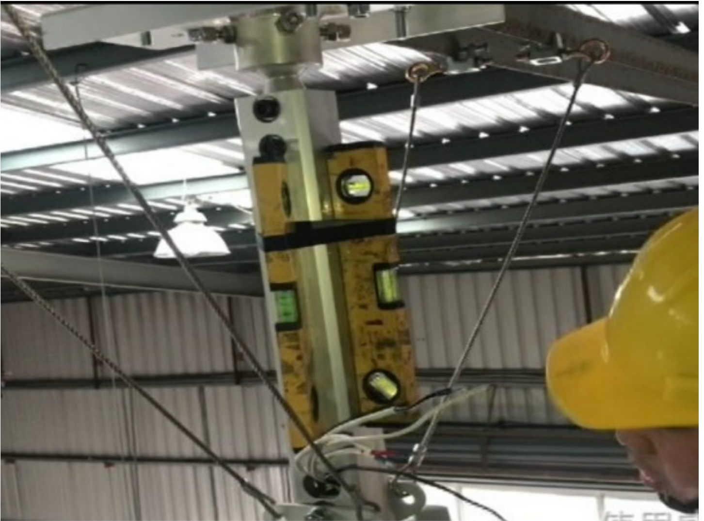
Diagram 15 (Completed guy wire installation):
