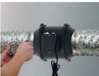
Attach the ducts with clamps.
