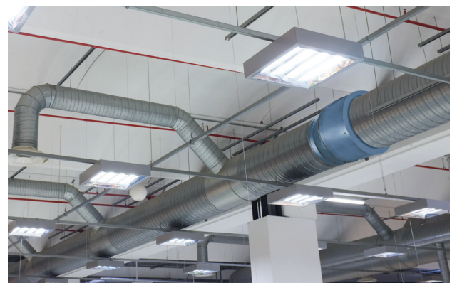
Ventilation example based on VKM fan
